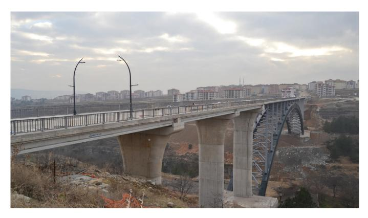
The intermediate supports of the new bridge are small enough to impose no limitations on the surroundings. The supporting columns of the truss bridge and the approach bridges are integrated into the inclined ground profile of the embankments. The superstructure is supported by a welded structure made from tubular steel with composite rectangular cross-sections. The horizontal and vertical main support tubes have a square cross section of 450 x 450 mm. The diagonal tension members.
